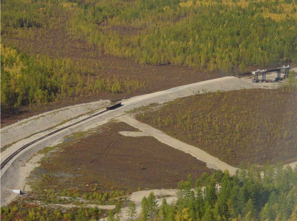
Figure 4. End of Rail Construction as of September 2005
